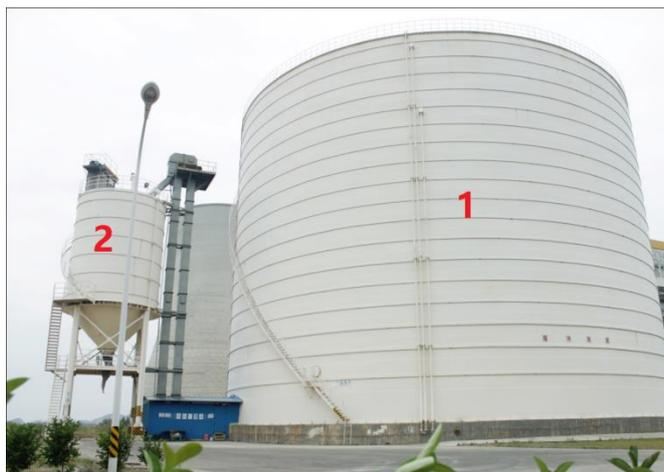
Picture 3. (1)Ash Storage Tank and (2)Surge Bunker
