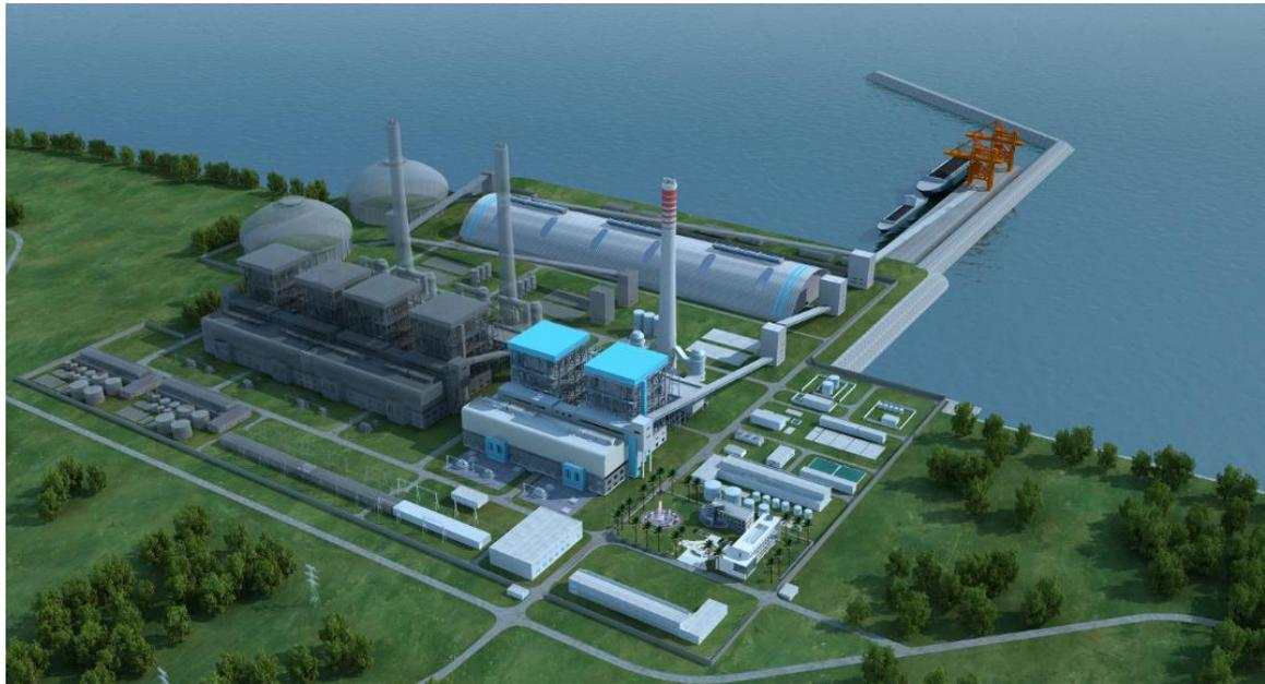
**Figure 3-1 General Layout arranged with the western area being the fixed end while the plant area would be extended.**
